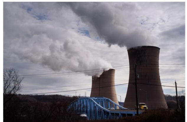
The Beaver Valley nuclear facility in Pennsylvania. PHOTO: JUSTIN MERRIMAN/BLOOMBERG NEWS Source WSJ, 01/07/24
